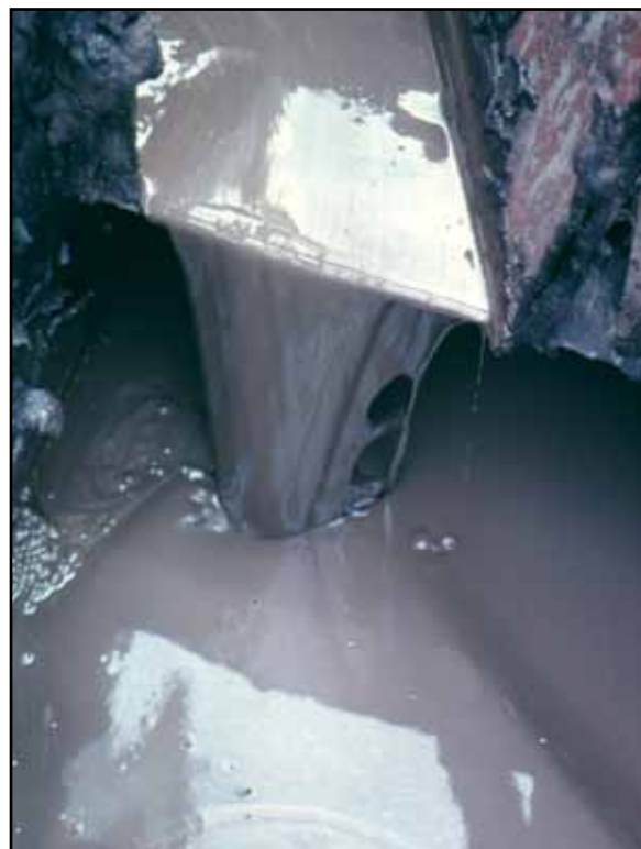
Figure 38. Drilling mud is a special liquid essential to the drilling process.
