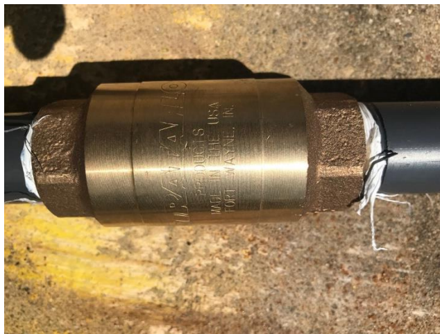
Figure 9 - Air Pathway Check Valve
