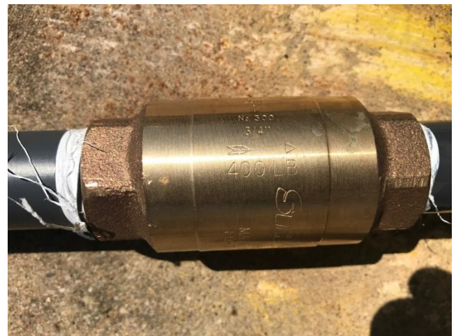
Figure 9 - Air Pathway Check Valve
